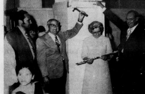
JOHN McCLELLAN, Administrator of Walker Memorial Hospital, watches as Dr. and Mrs. Larsen and Steven Pardee removes the first pieces of wood from the original building of Walker Memorial Hospital that is to be demolished in the near future. Photo by Sharpe
