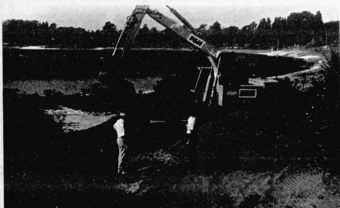
TUESDAY MORNING TRI-SURE Corporation back-hoe operator, Johnny Mech moved the first dirt for the North Lake sewer extension lift station on Lake Isis Drive. Watching are Mayor Marshall Davis, and O. K. Mock, manager of the corporation, utility division. Sunphoto by Lew Miller.
