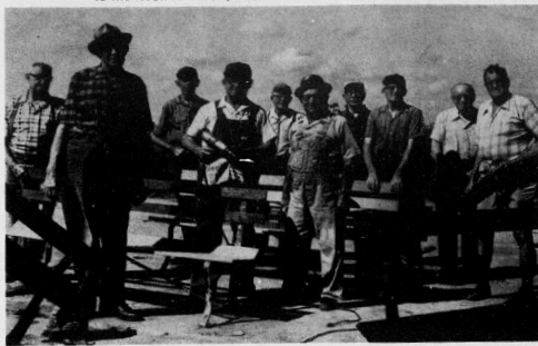
ONE OF THE COMMUNITY PROJECTS of the Avon Park Grange, was the repairing and painting of the benches located along our "Mile Long Mall". Pictured above, from left, are Alfred Haviland, Edwin Swanson, Keith
