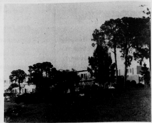
PART OF THE NEW addition to Walker Memorial Hospital can be seen through the trees from the South-West side, (Lakeside).
