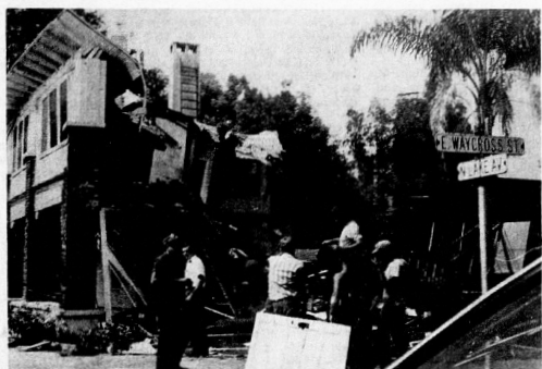
ONLY THE FRONT wall stands on this old landmark, and that piece of the building came tumbling down minutes after this picture was made, as the wreckers demolished the historic Poinsettia Hotel last week. The building had stood at the corner of Waycross Street and Lake Avenue since the late 1890's, but in a few more weeks the site will be an additional parking area for customers of the Avon Citrus Bank. Photo by Sharpe
