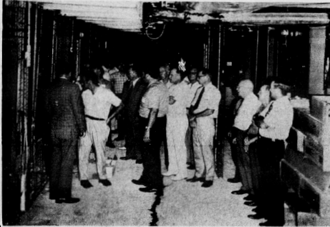
BY STAYING OUT of the hard hat or working areas, Avon Park Rotarians, under the leadership of John McClelland (center) Hospital Administrator, were taken on a tour of the new addition to Walker Memorial Hospital. They paused to look at uncompleted rooms and overhead con ducts for air conditioning, electrical, water and heating.
