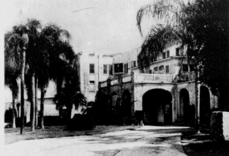
THIS OLD 1920 building will come down sometime within the next two years following construction of the new Walker Memorial Hospital structure. Groundbreaking ceremonies took place at 11 a.m. Wednesday morning. The
