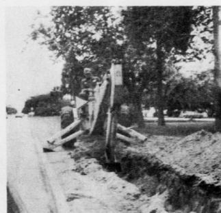
MALL BEAUTIFICATION - Shown above is a city employee busy working on new underground irrigation for Avon Park's famous mile long mall. The ground along the curb had built up well above the curb and was destroying the grass. The city removed the excess soil, and is presently placing in new plastic irrigation pipes along this area of the mall. Work is expected to be completed within a week. (Photo by Neil Williams.)
