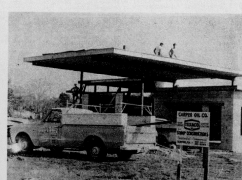
MORE PROGRESS in Avon Park. This $45,000 new Texaco service station under construction on Hwy. 27 south of Avon Park, is scheduled to open the middle of January. A modern Texaco
