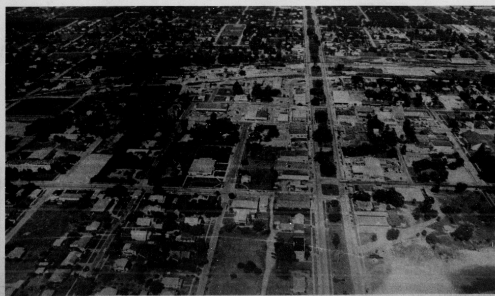
AERIAL VIEW OF AVON PARK
