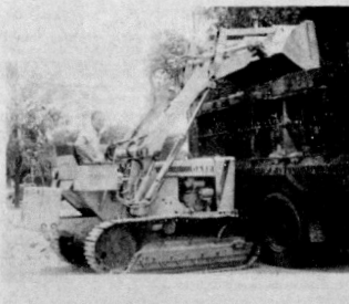
EMPLOYEE of Maurice Albritton, contractor, is shown loading up gravel and dirt at the site for the new building of the First Baptist Church Monday afternoon after ceremonies.
