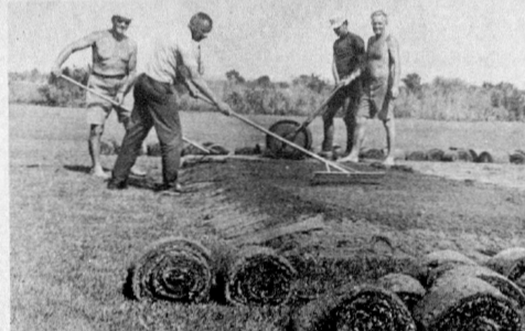
JOE GROH, Ross Hendrick, Rodney Davis and Tommy Bagwell work on the new 6 Tee at River Green Golf course in preparation for the Bagwell Lumber
