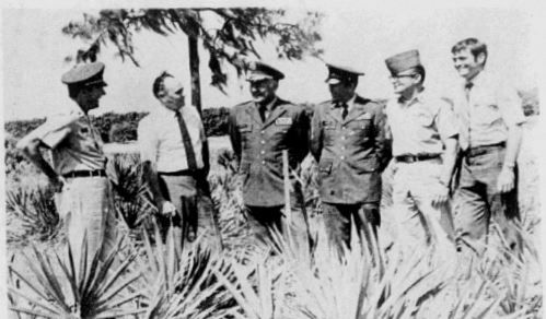
THIS GROUP is shown looking over the site for the new National Guard building. Funds have already been appropriated and plans are being finalized with construction to start in the near future. The site is located just south of Avon Park on US 27. Left to right, Warrant
