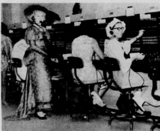
CLOETTE WITTEN, Mittie Barnes and Bea Jones at switchboard at the Telephone Co. last Friday.
