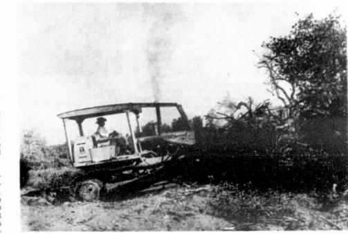
JAMES "BUDDY" McROY pushes trees in to the fire at the site where the new high school will be built on the Bomb-
