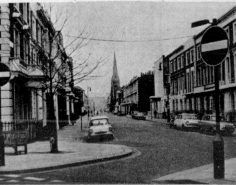
LONDON'S ANSWER to speedsters swerving and careening through quiet neighborhood streets. Wide streets give way to very narrow bends at each corner. Speeders soon tire of accelerating when they have to apply brakes quickly to make turns.
