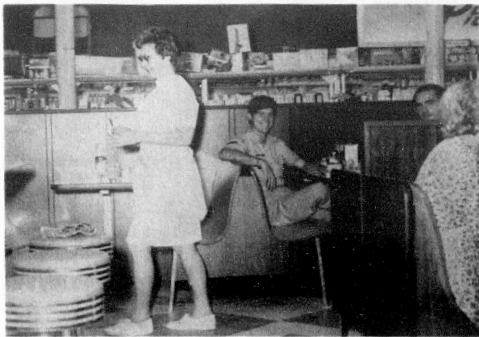
PICTURED ABOVE is a section of Touchton Drug's which is undergoing a complete remodeling. Shown is "Marie" one of the favorite waitresses at the serves
