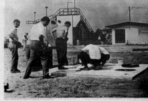
FINAL INSPECTION and trial operation of the lift station at the South Florida Junior College was held on Sept. 4. Left to right: an employee of J. I. Newton Utility Construction Co.; City Councilman, Russell Scott; F. R. (Bud)
