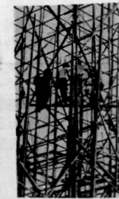
LOOKS LIKE modern art, but it's really just construction men standing atop huge bamboo poles, part of a structure being erected for a fair in Hong Kong.
