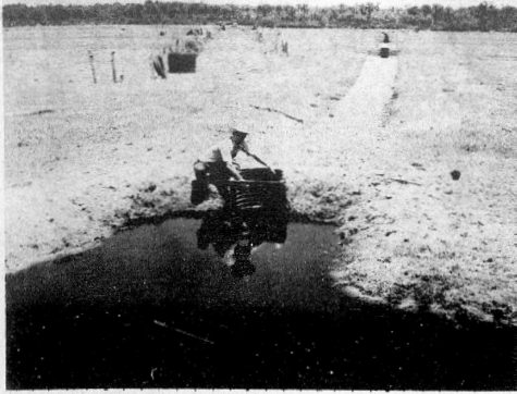
CONTRACTOR GRADY MERCER of Sebring puts finishing touches to water control system for improved pasture on the Henry Perry Ranch Southeast of Lake Placid.
