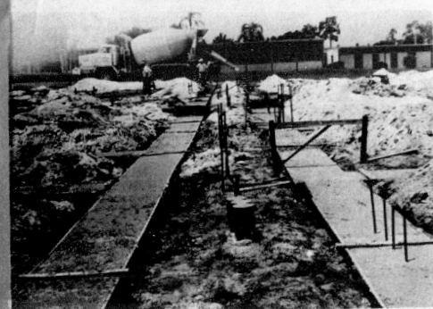
WORK IS UNDERWAY on the new $188,000 educational-treatment building at the Florida Alcoholism Treatment and Research Center in Avon Park. Structure was designed by James A. Heim.
