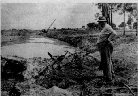
THE CANAL shown here being cleaned out runs through the golf course from Lake Damon to Trout Lake. When com-
