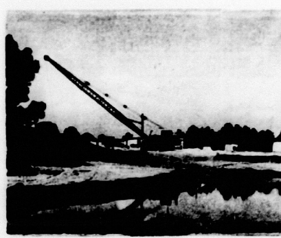
EXCAVATION is underway on the site for the SFJC being built on the shores of Lake Glenada, south of Avon Park.
