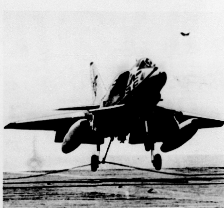
A CRUCIAL SPLIT SECOND is captured by a photographer aboard the carrier USS Hancock as an A-4 Skyhawk, world's smallest attack bomber, catches the No. 1 arresting cable while landing after a mission over Vietnam.
