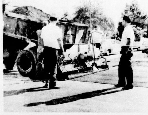
SPACE TO PARK is being provided at the Bagwell Lumber Company for its customers as the former packed sand surface is being replaced with a mac-
