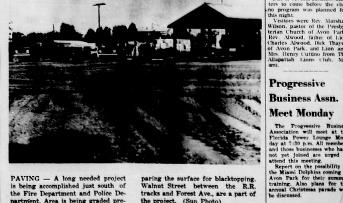
PAVING — A long needed project is being accomplished just south of the Fire Department and Police Department. Area is being graded preparing the surface for blacktopping. Walnut Street between the R.R. tracks and Forest Ave. are a part of the project. (Sun Photo)
