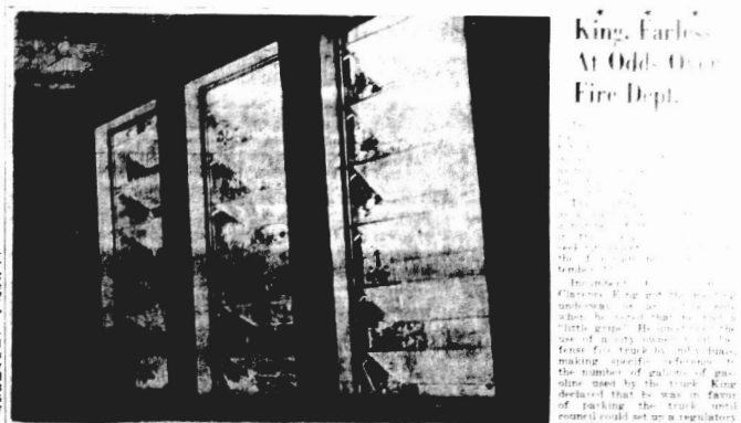
NEW CITY HALL WINDOWS—Workmen were busy this week installing new awning type windows in the Avon Park City Hall. The windows relieve the problem of heat, one councilman said and at the same time enhance the beauty of the building. Most of the installation work was done by city employees. (Photo By Sun)
