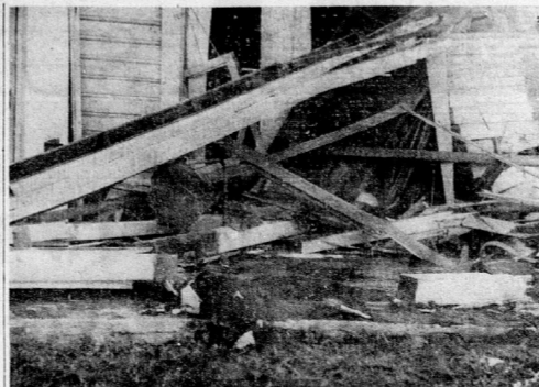
THE H. C. GARRETT home on South Verona Avenue after being hit by a truck last Wednesday. The driver crashed into the house demolishing the living room and damaging furnishings. The family was uninjured in another room of the home. The driver was later arrested after abandoning the truck at the foot ball field, and was charged with leaving the scene of an accident and driving without an operators license.
