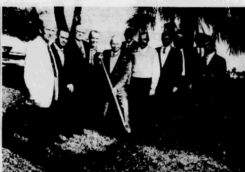
LAKE ROSALIE, FLORIDA—Shown here turning the first spadeful of dirt for the construction of a $385,000 clubhouse for the Tiotie Beach Yacht and Country Club is Col. James E. Huffman, Commodore of the Tiotie Beach Resort and a partner in the Tampa firm of Schulstad and Huffman. Others, left to right, are: Polk County Commissioners J. B. Thornhill, Jr., Alfine Conroy, Roy P. Gladden and E. A. Largent, Polk County Engineer Lawrence Lohr, Edward L. Bolding of the contracting firm, Le and Lowe, Executive Director for the Tiotie Beach Yacht and Country Club, Joe Boye and Bill Meyer, Editor of the Avon Park Sun.
