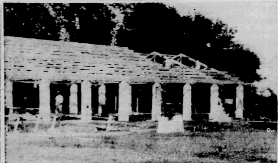
EXPANSION PROGRAM FOR EXPOSITION Workmen are rushing to completion the new livestock pavilion at the Hardsee County Cucumber Exposition grounds to have the building ready for the opening of the Exposition, which will get started Nov. 9 and run for six days. The new exhibits of halter broken cattle and poultry will complete the agricultural picture of the Peace River Valley Area at the Exposition which already features citrus and produce. The Exposition has grown from a "tent show" to the present spacious grounds with modern exhibit buildings in 13 years, and the expansion program now in progress will make it one of the outstanding agricultural events of South Central Florida.
