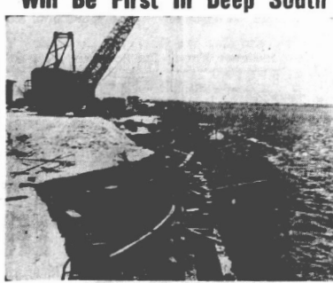
SOON TO BE COMPLETED near Jacksonville, Fla., the big Mayport Carrier Basin will be the only harbor facility between Norfolk and San Diego large enough to accommodate the Navy's big aircraft carriers.
