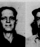
Hoyt P. Cannon Boiler Operator
