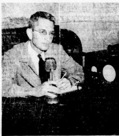
SHERIFF HAS NEW RADIO —Sheriff Broward Coker is shown at the controls of the new two-way radio system recently installed in his office for contact with patrol cars. The tower is shown at right.
