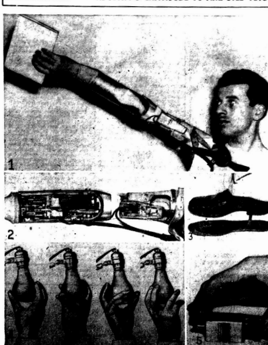
While it will not be available for some time, this electrical arm and hand (1) has been developed by International Business Machines Corp. in cooperation with the Veterans Administration. IBM announced the development as a token of gratitude to amputee veterans. The electric mechanism is housed in the forearm (2) and arm movements are controlled by pressure upon pneumatic bladders (3) under the big toe. The arm and hand make almost all the natural movements of the human arm and hand, and some the latter cannot. The nylon hand (4) can be rotated continuously at the wrist. A $15,000 electric motor (5) occupying 2 cubic inches was designed for the arm. Power is supplied by a battery, then can be recharged overnight.
