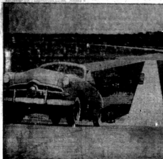
NEW FORD TEST HILL —This 1942 Ford is climbing the 30 per cent grade on the new test hill at Dearborn, Mich., which was constructed of 124,000 tons of steel slag from the Ford Motor Company's steel mills. This 30 per cent grade approximates San Francisco's famed Filbert street—long a favorite among test engineers as one of the steepest city streets in the country. Hill-climbing ability, automatic transmissions, foot and hand brakes, bumper clearance and carburetion are tested on the new hill by Ford engineers. In addition all Ford products are tested under extremes of temperature and terrain in all parts of the United States.
